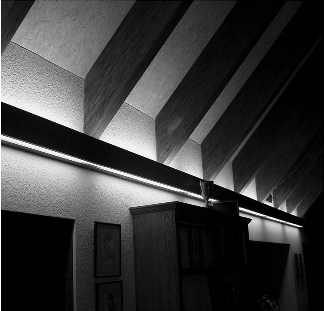
Figure 7.13 Photograph showing soffit lighting of ceiling rafters.
