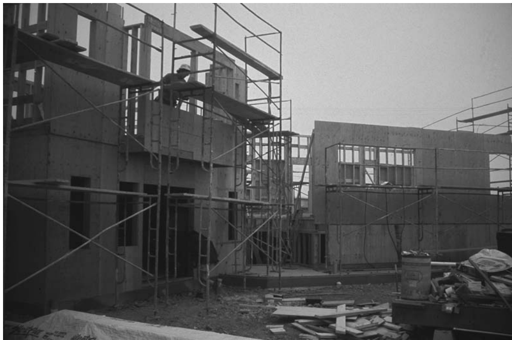
Figure A.4 Second floor walls nearing completion after tilt up.
