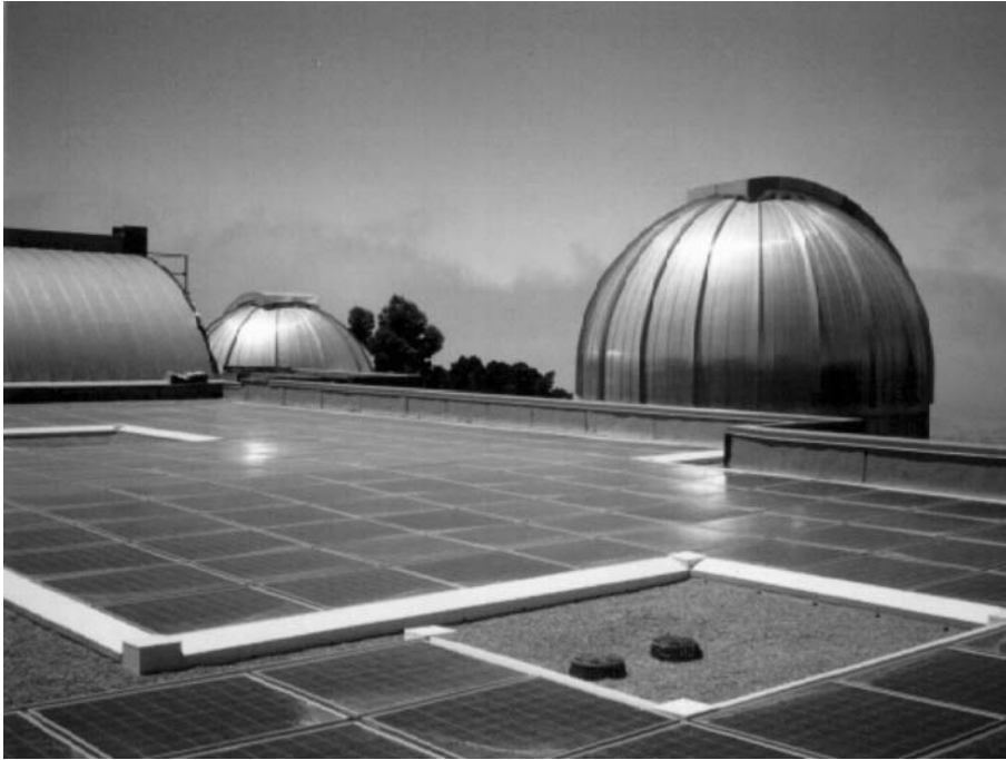
Figure 14.1 Powerlight foam solar PV collector roof tiles.
