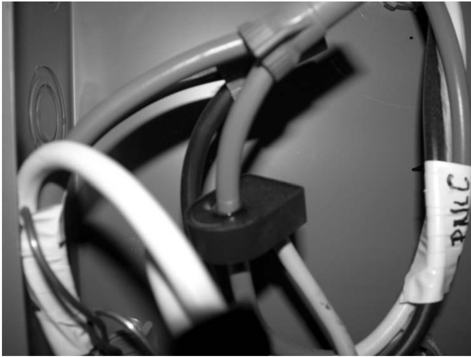
Figure 13.5 The current Toroid sensor.
